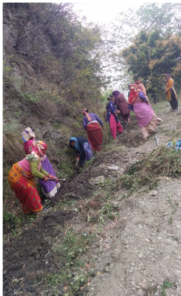
During Cleaning Canal at Pata
