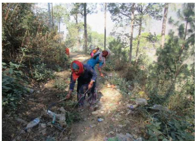
During Cleaning Canal at Pata
